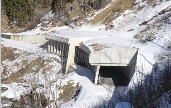
Avalanche and rockfall protection
