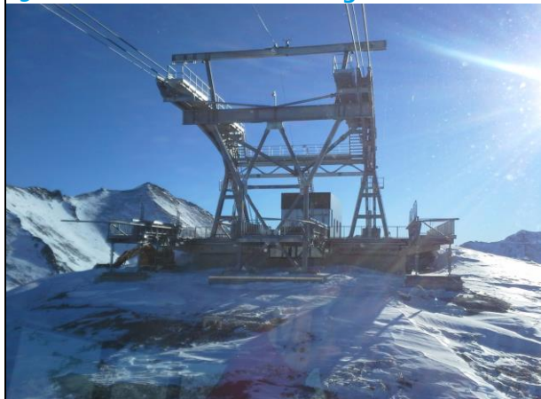
Top station finished
