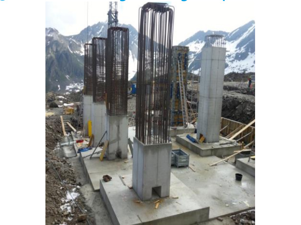
Single foundations and lifting columns
