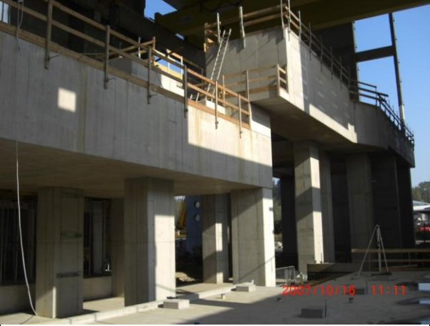
Complete turbine foundation finished
