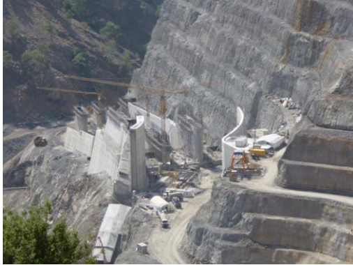
Detailed view during construction
