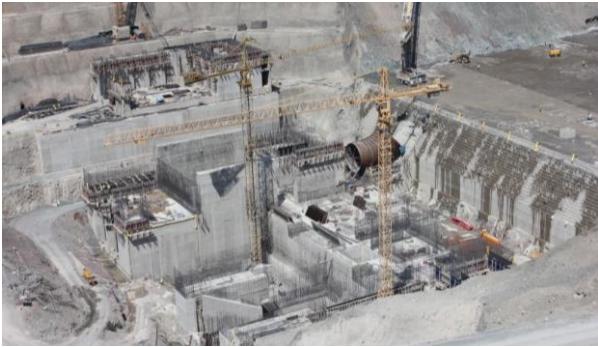
Detailed view during construction
