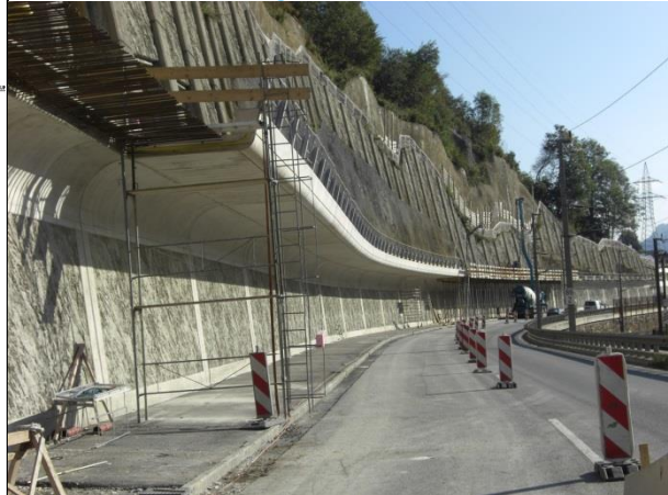
Protection of walkway and highway
