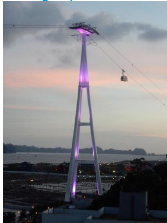
Highest cable car tower in the world 188,88m!
