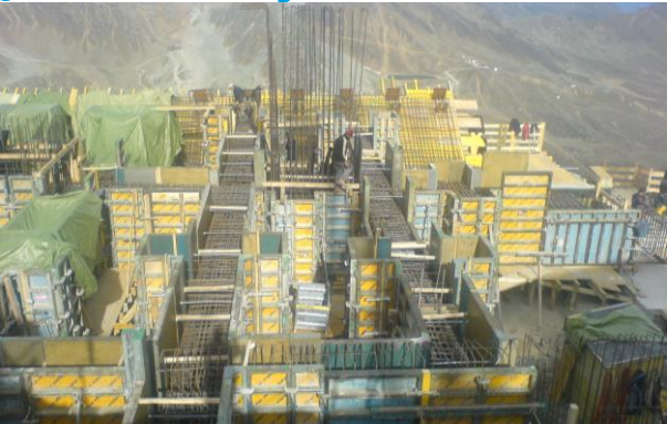
Top station: Truss beams under construction
