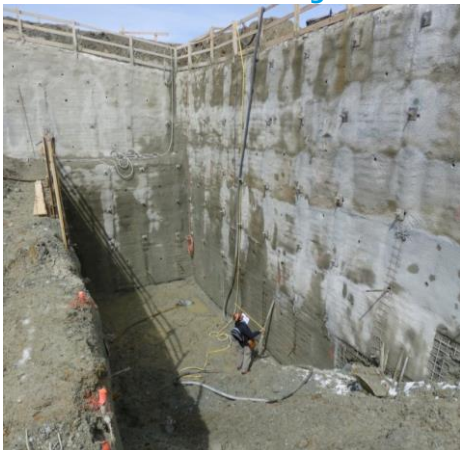
Top station: Permafrost unfreezing during excavation and anchoring measures
