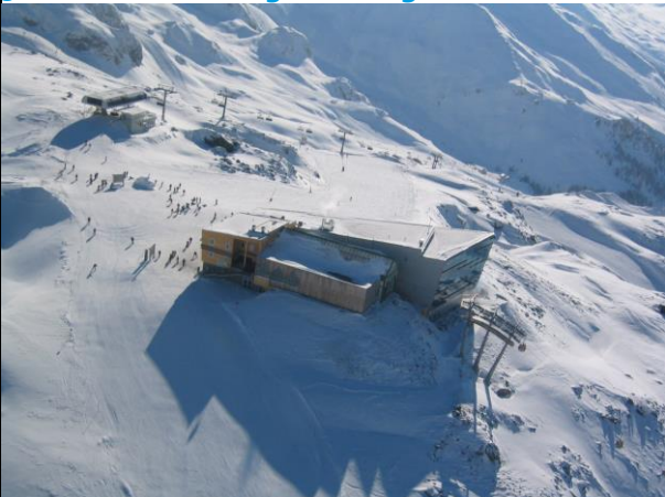
Area of new Top station and Tower 5
