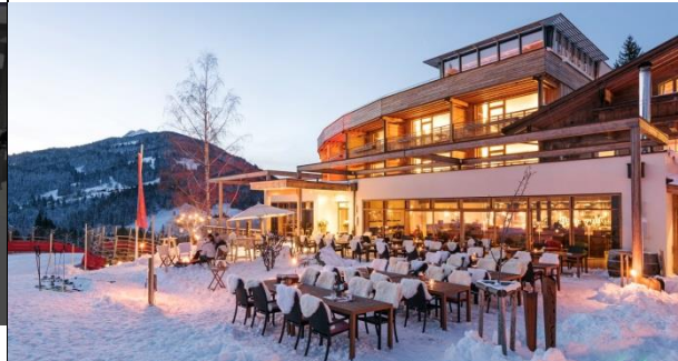
Complete hotel in wood structure
