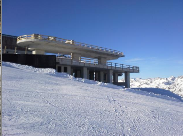
Concrete structure finished
