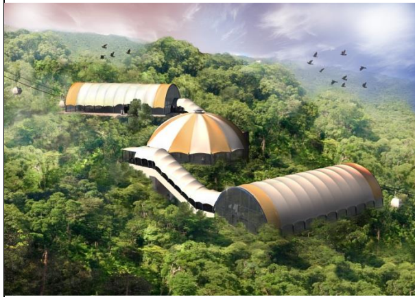
2 cable car stations and distribution building
