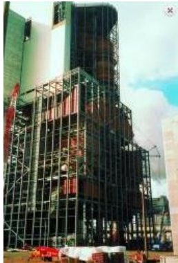
Boxberg – Luvo- and coal bunker house
