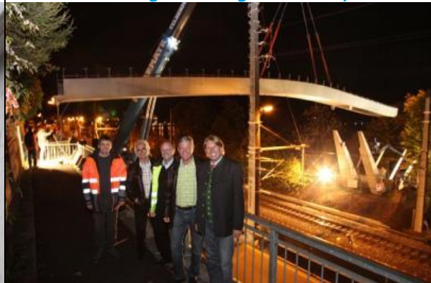
Heldenhain bridge crossing the railway lines
